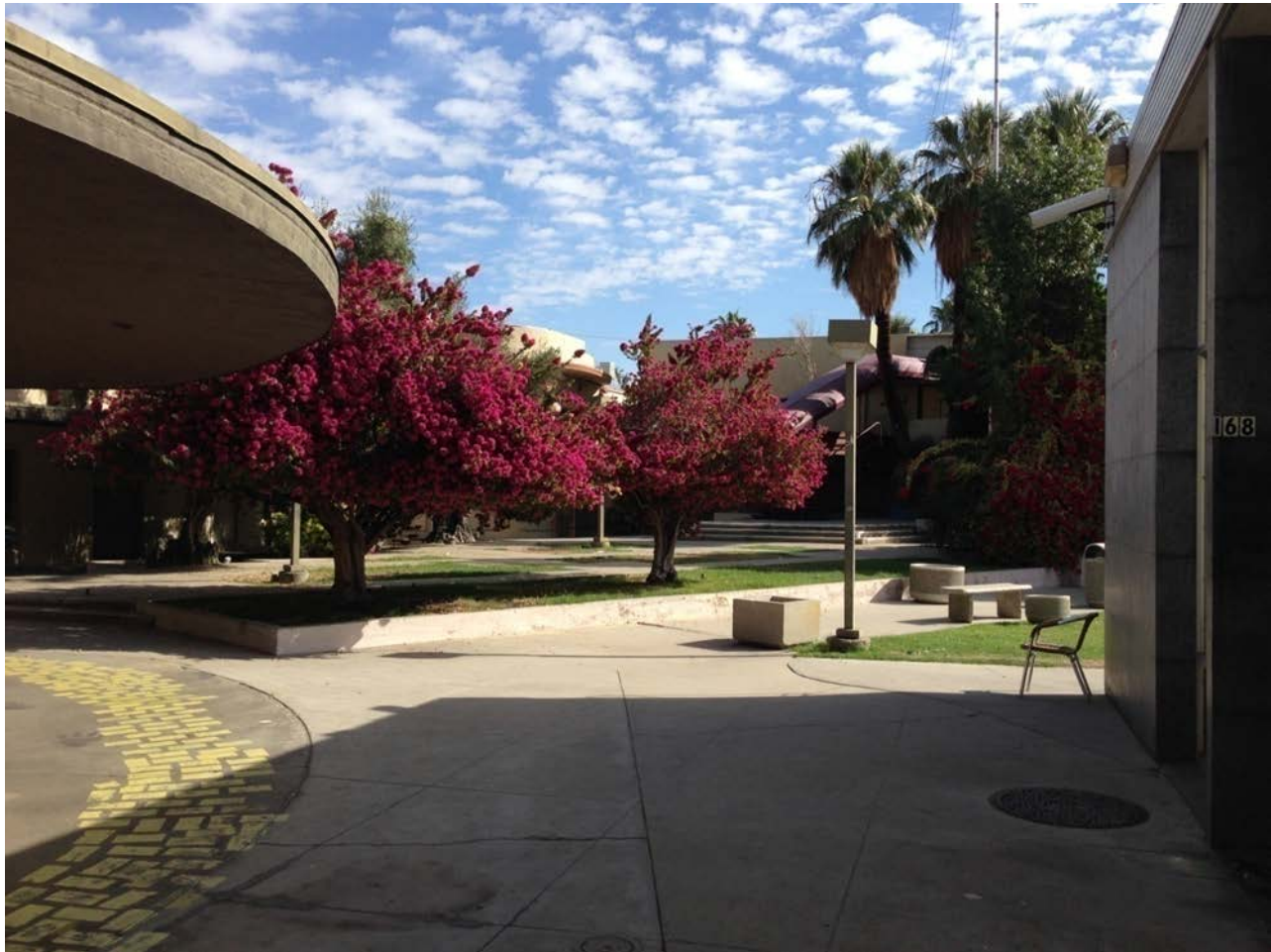
Photo 6. Approaching courtyard, looking east, with Building A (Twin Building North) in the foreground at left; across the courtyard is the rear portion of Building A , and Building D (Town & Country Restaurant), Building E at right, May 2014
