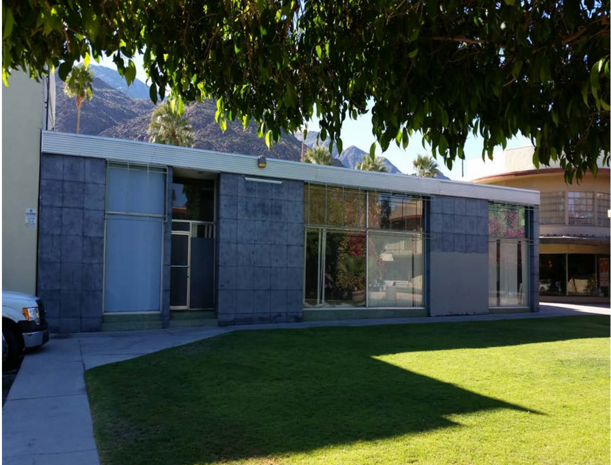
Photo 11. In the courtyard looking west toward Building E with Building A in background, March 2015
